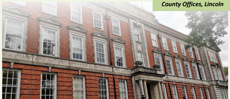
County Offices, Lincoln
